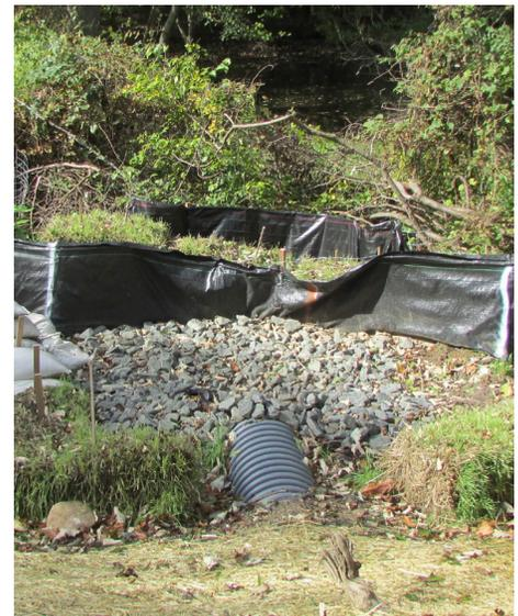
Wetland being comprised – Featherfoil pond now silted as water went though and underneath fencing
