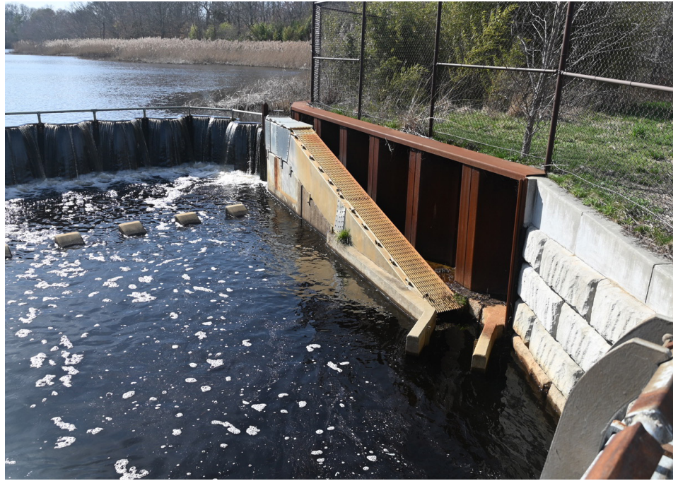
The fish passage on the Peconic River, near River Road in Riverhead. Photo: Byron Young
